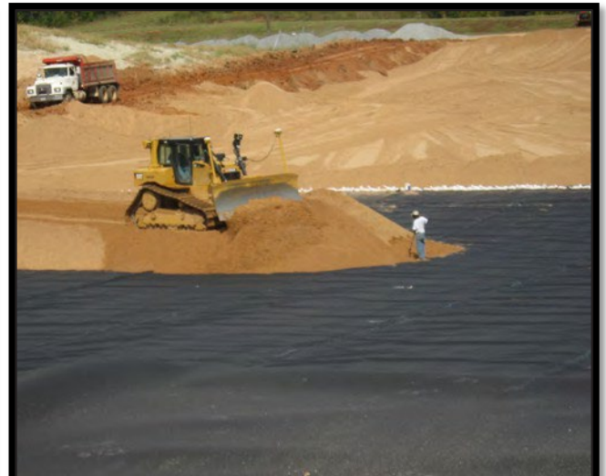
Placing Protective Cover
