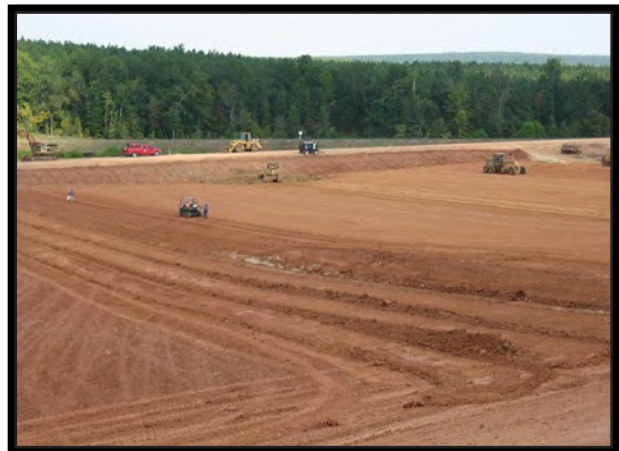
Phase IV Cells 3, 4 & 5 Construction
