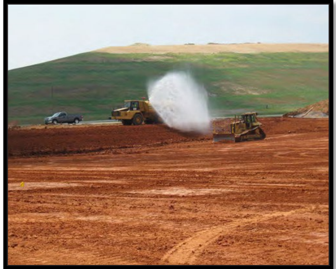
Applying Water To Clay Liner
