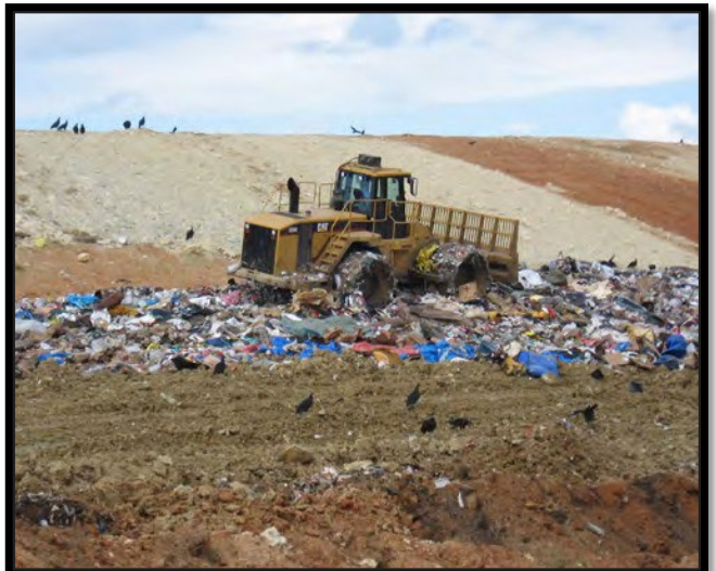
Compactor Working Waste
