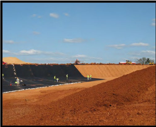
Liner Being Installed
