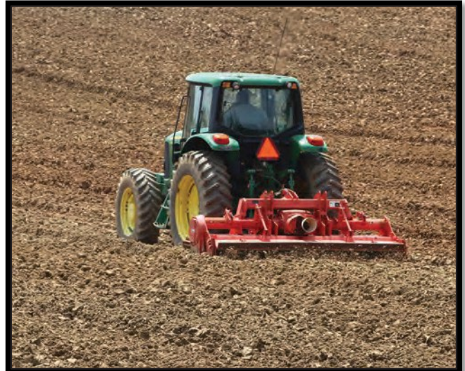
Processing Soil For Clay Liner
