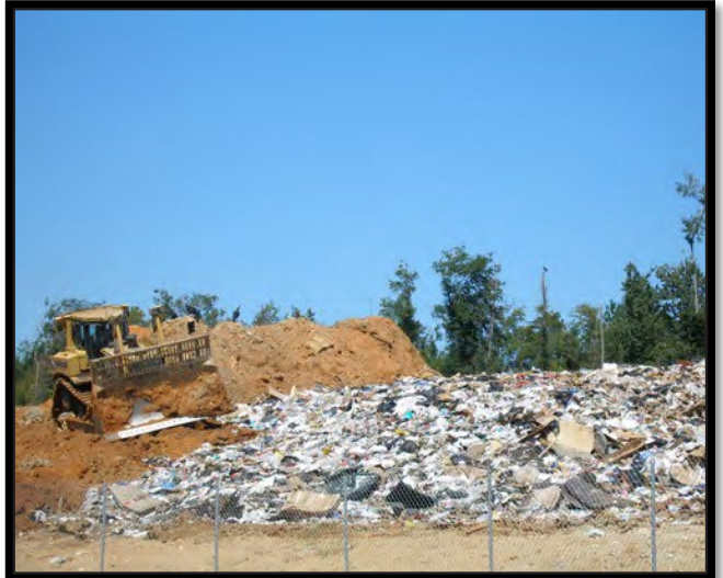
Waste Being Covered Daily
